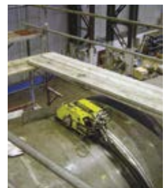
Trav-L-Cutter being used for submarine decommissioning
